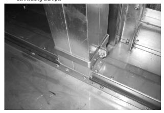
Finally, seal the separation point of the unit parts on the inside with the sealing compound supplied.
