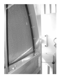
As a matter of principle, the bearing of the rotor is aligned in the factory. However, depending on the installation conditions, a realignment may be required. Please refer to the manufacturer's operating instructions.
