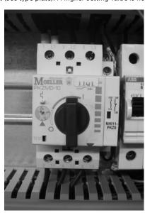
Protect motors with built-in PTC thermistor sensor using a PTC thermistor tripping device.
