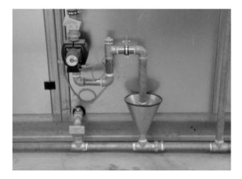
Horizontal drain pipes must have sufficient diameter, slope and ventilation and venting for trouble-free water drainage.
