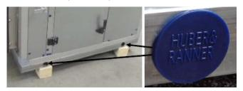
Intermediate base frames that are in the air flow must also be sealed on the inside with the blue cover plugs.
